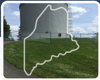
Basic Public Infrastructure
